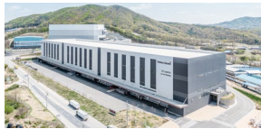
Yongin Logistics Park 1 GFA 70,028m 2 | Completion 2017.11
